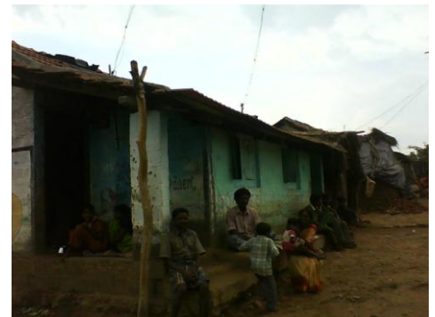
Two defunct houses constructed under tribal settlement project by the forest department in 1995 [B.Matakere GP].
