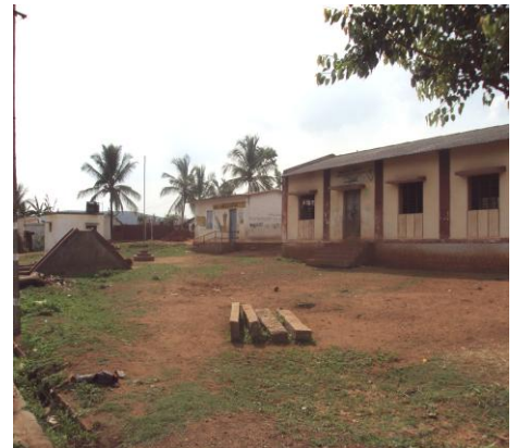
A shed constructed by government to carry economic activities by the tribal community.
