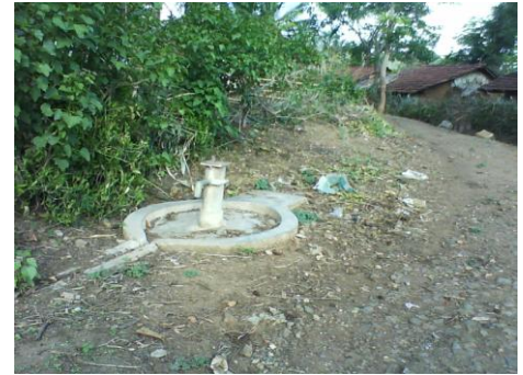
A bore well where the pumping hand is removed by unknown people in N.Begur GP
