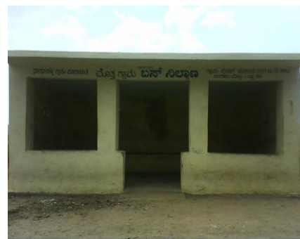
Construction of a Bus shelter in Naganahalli GP.
