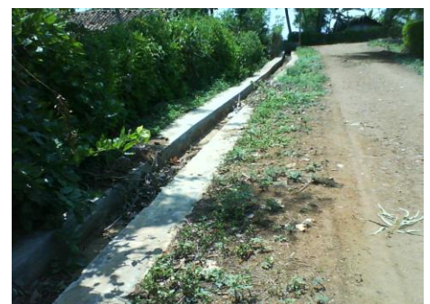
Two drainages constructed under government scheme in N. Begur GP.
