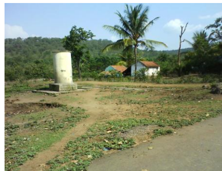
MWS tank in N. Begur GP
